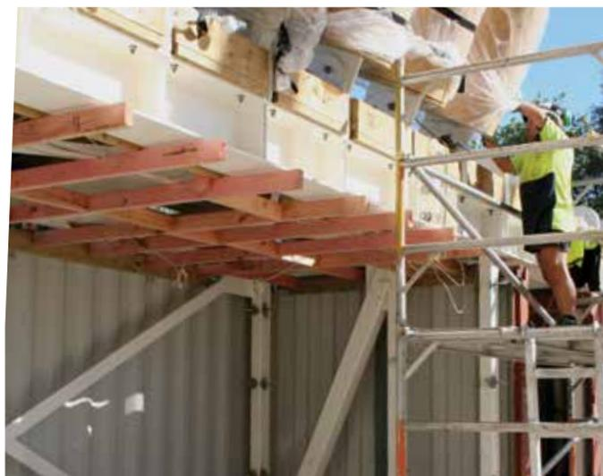
Bottom: Naylor Love Construction fixing the base connection of the cardboard rafter to the container steel. Every connection is at a different angle and each rafter has been 3D modelled throughout the building to allow set out of the flare. The container fit-out and structural steel is also visible.
