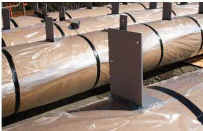
Middle: Detail of the cardboard rafters prior to lifting in place on site. Each of the cardboard cores is manufactured off site, purlin cleats attached, and wrapped in plastic sheeting to reduce water and handling damage.
